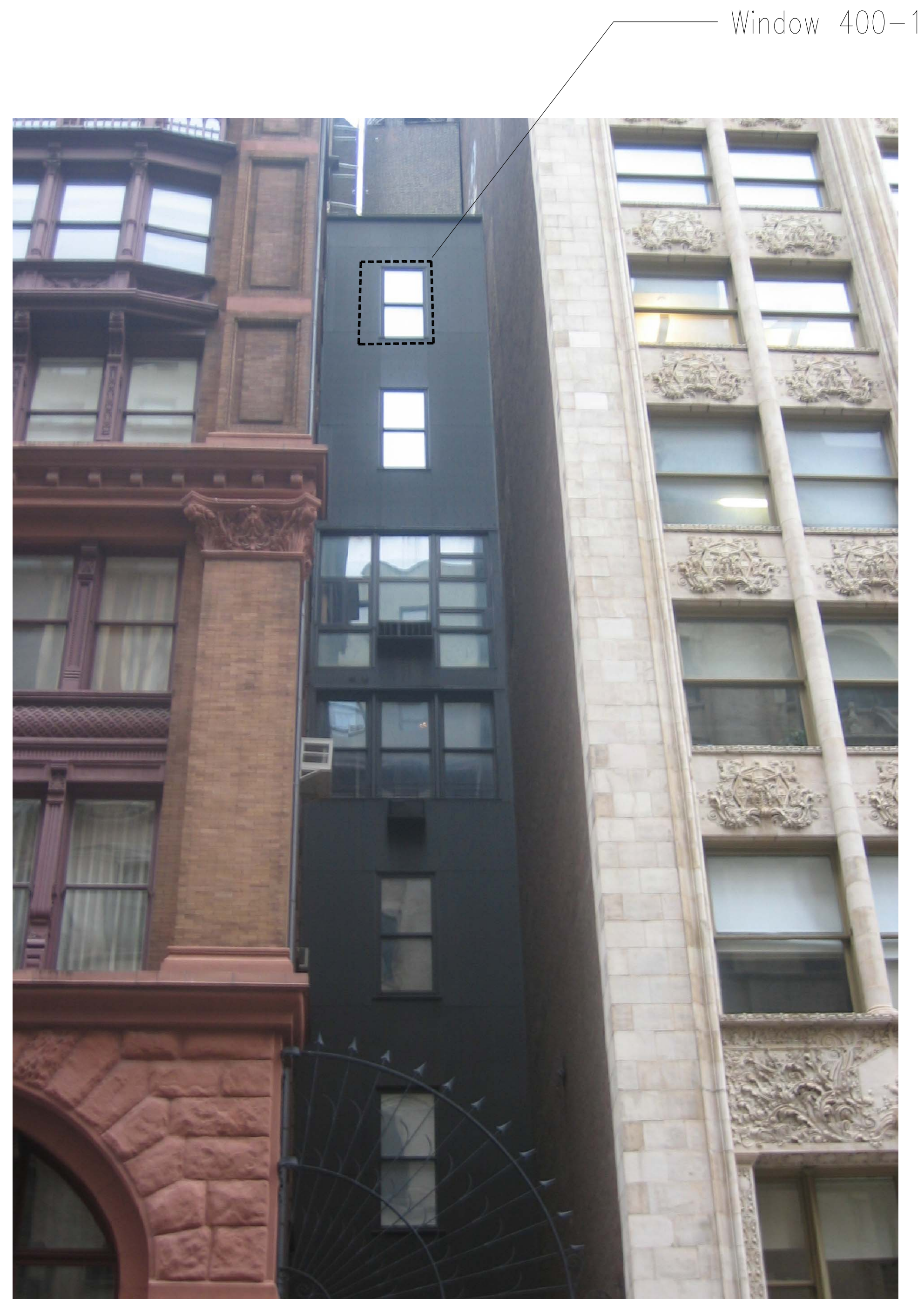
3 South Facade - Existing Condition no scale
