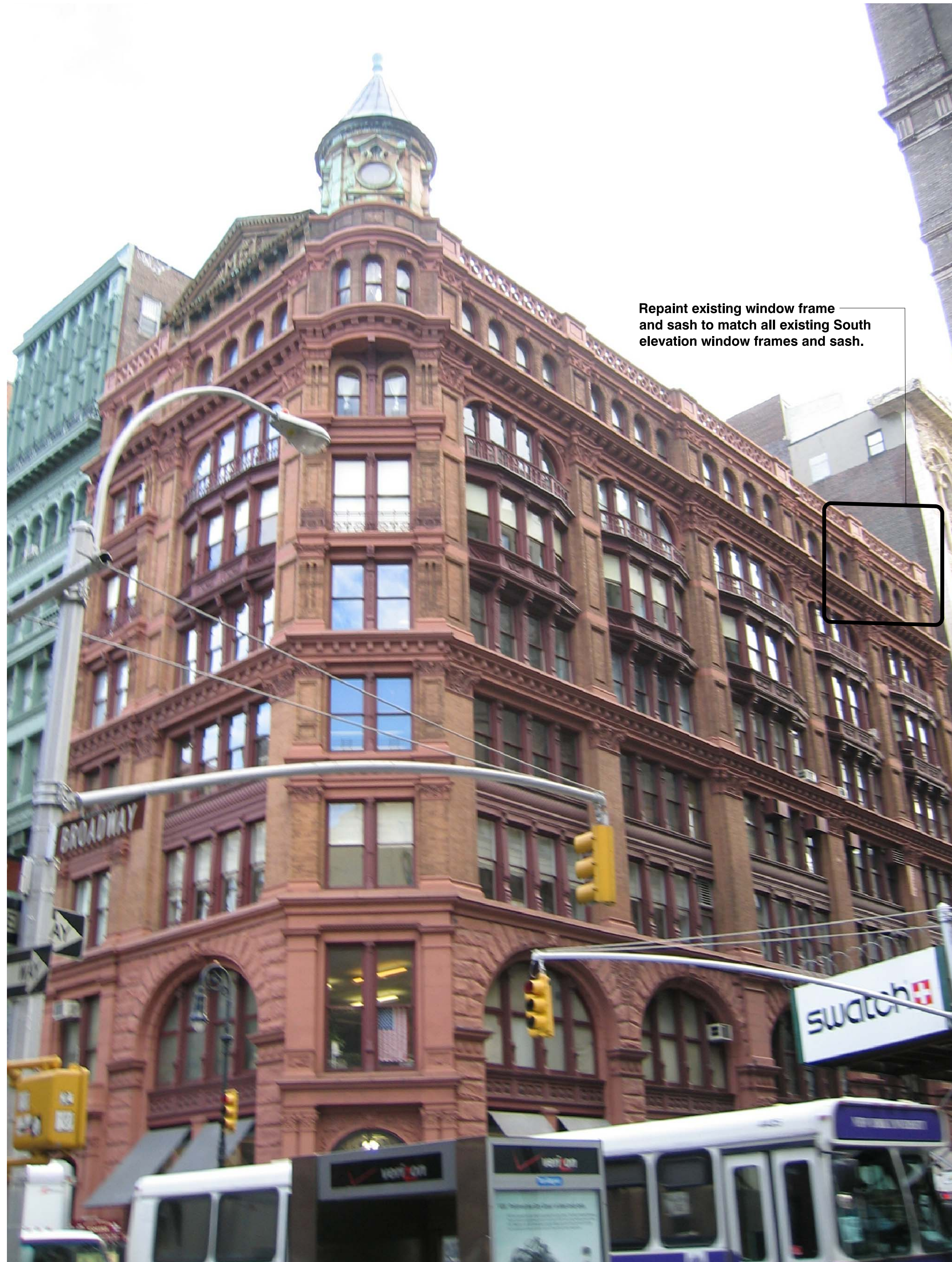
Looking Northeast at the corner of Broadway and Bleeker
