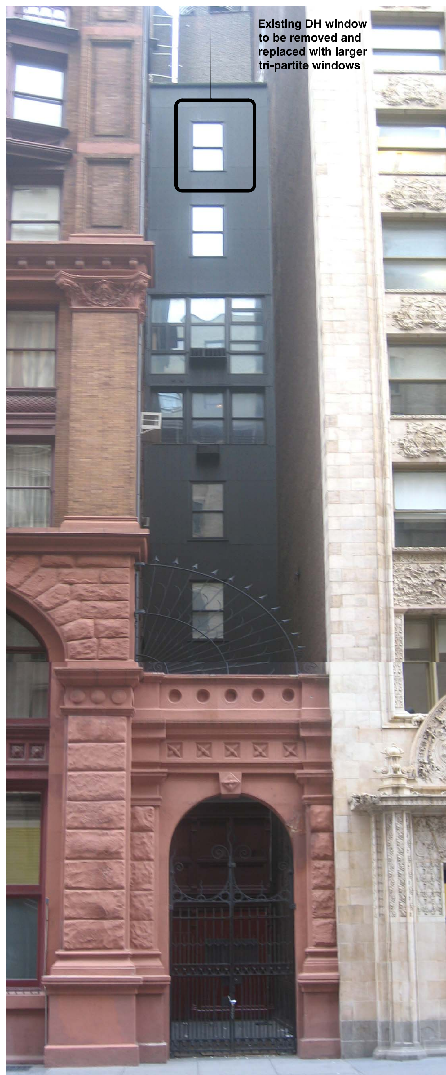
Looking North at set back on Bleeker
