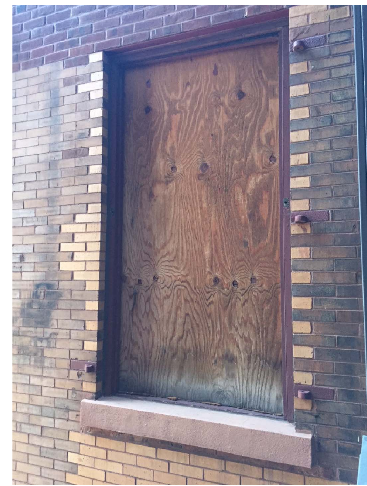
3 Window 300-1 Existing Condition no scale
